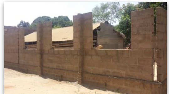
Permanent building under construction in Kibaha near Dar es Salaam.
